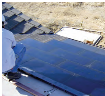
Open Energy solar panels being installed
